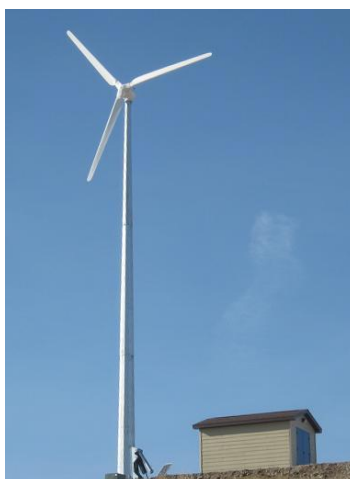
Fig. 3.9. REDriven 3 KW wind turbine with three blades,
