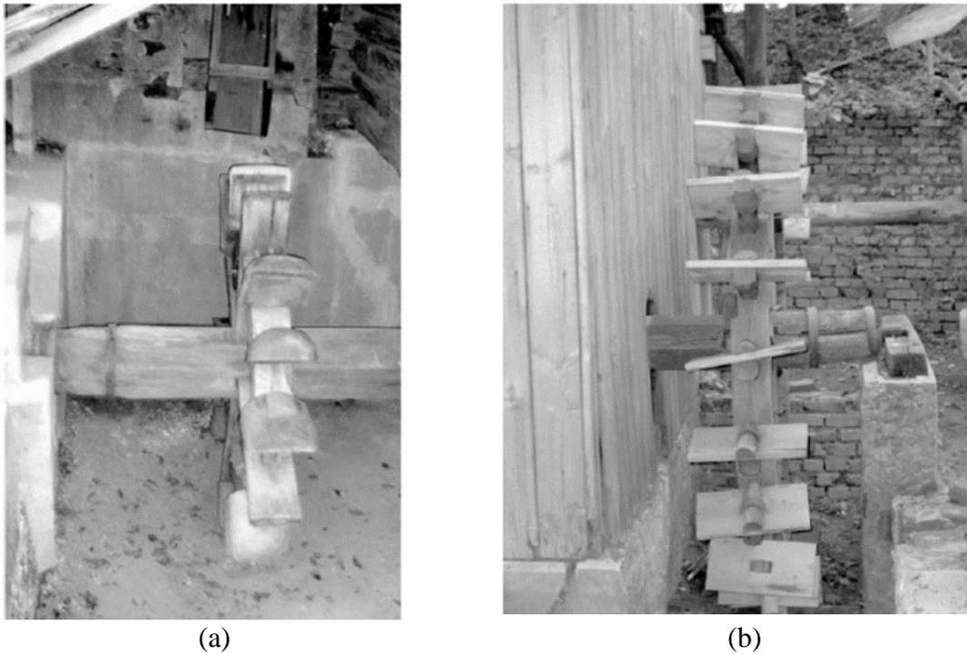
*Figure 1.5 - Water wheels with action [Village Museum, Bucharest]: (a) rotor with straight blades; (b) rotor with buckets and inclined gutter directing the water jet towards the buckets.*
