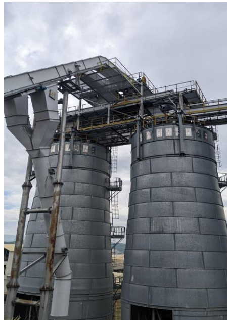
Figure 8. Current 500-ton silos of the Alfa Wood Nevrokopi Company
