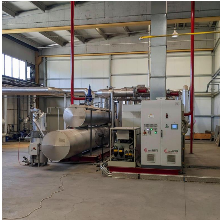
Figure 2. Alfa Wood Nevrokopi's Turboden ORC cogeneration systems
